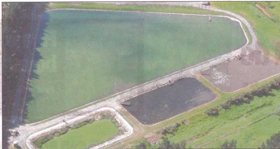
Taipā's wastewater ponds in the grip of an algal bloom in December 2017.
